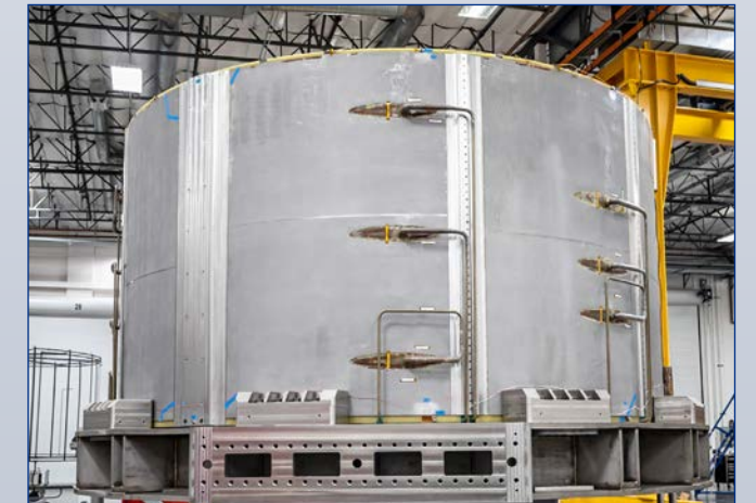
Module after piping installed
