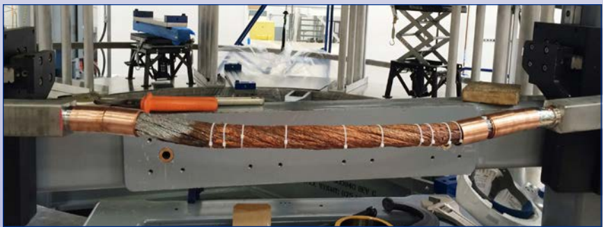
Splicing the conductor cable together similar to splicing a rope
