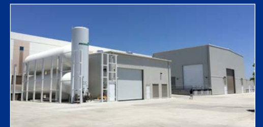
Final Test Facility
