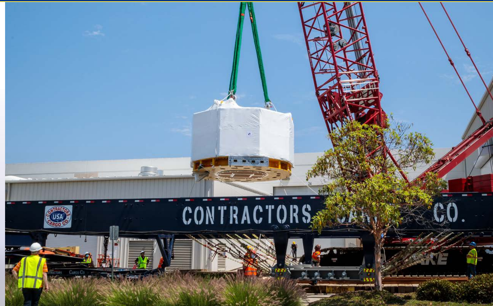
Lowering module into the 24-axle super-heavy trailer
