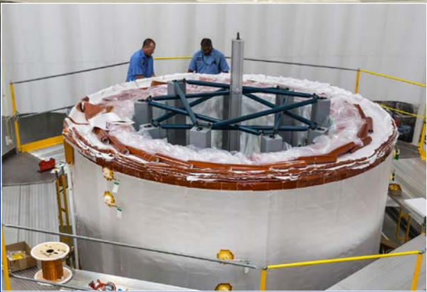
Module during ground insulation application
