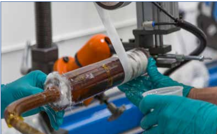
Thirty-nine helium pipes welded and insulated to provide the supply and return for supercritical helium at 4.7 K
