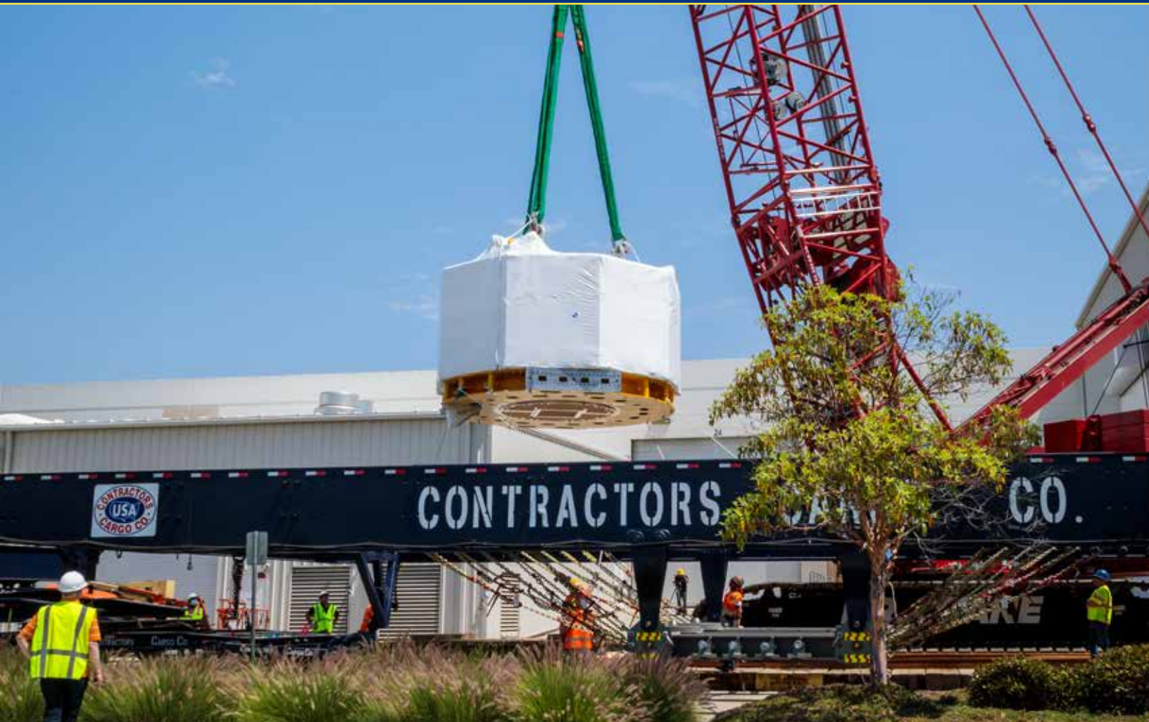
Lowering module into the 24-axle super-heavy trailer
