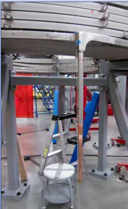
Terminal lead nearing completion
