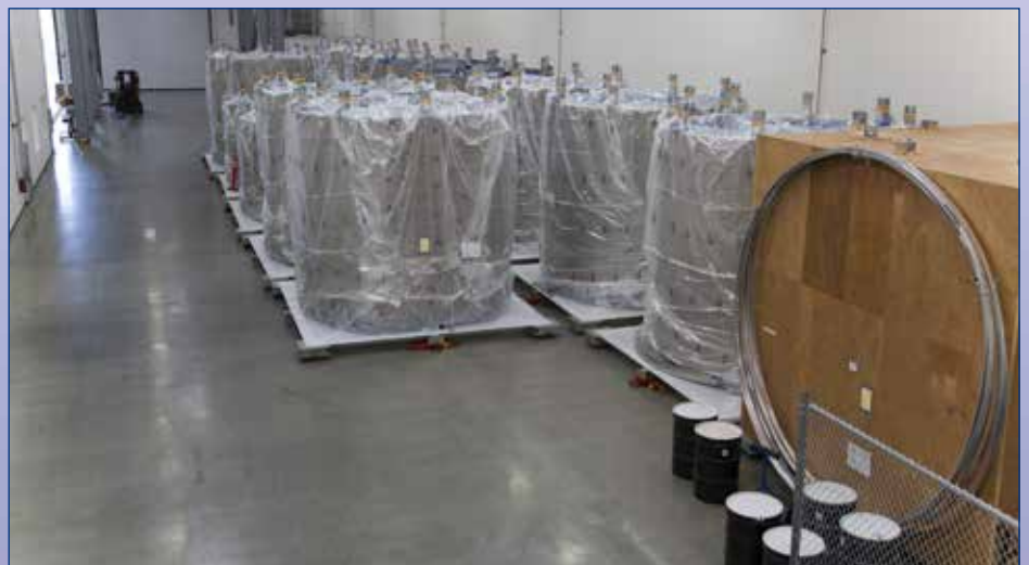
Conductor spools stored prior to winding
