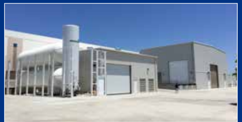
Final Test Facility
