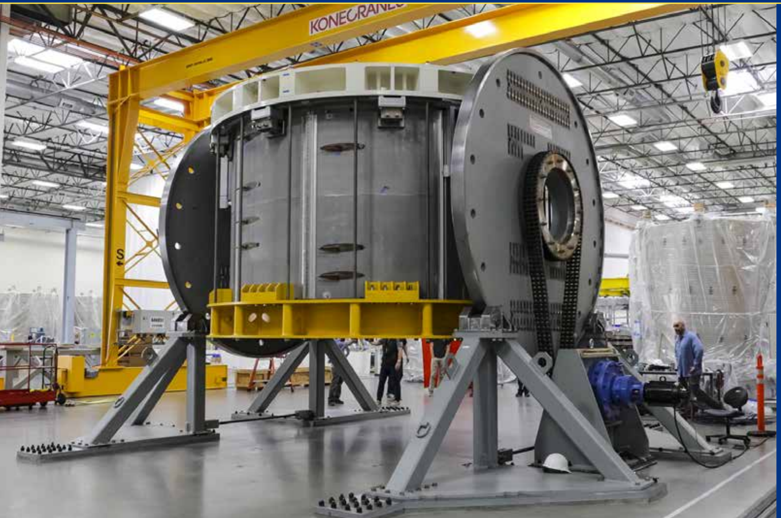
Modules require rotation to exchange bases under coil and allow access for piping installation
