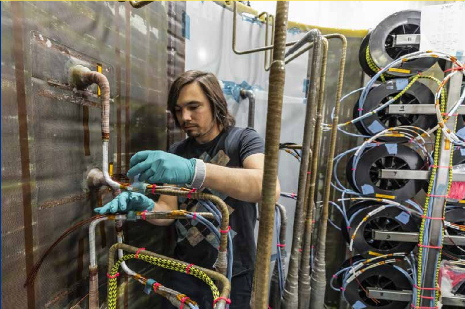
Technician applying insulation to piping on inner bore
