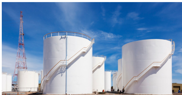
Figure 2. Slurry oil settling tanks.
